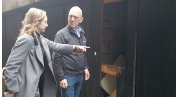
Claire-Louise, Leila and Steve inspecting the problem areas
